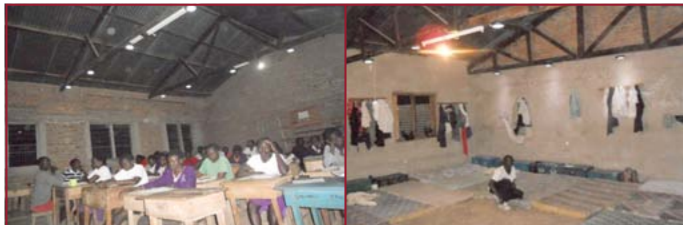
Time to work hard. Girls of Koboko parents using the installed light at night. One of the dormitories installed.
